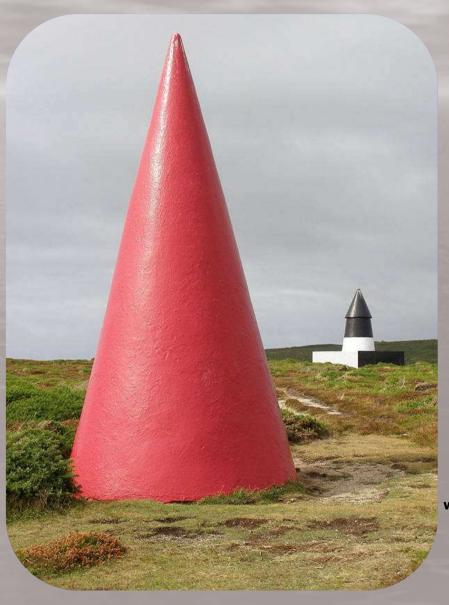
\*Actually, they're 'day marks', which provide a visual warning to vessels, of the extremely dangerous Runnel Stone reef, which is just offshore from the watch <sup>©</sup>
